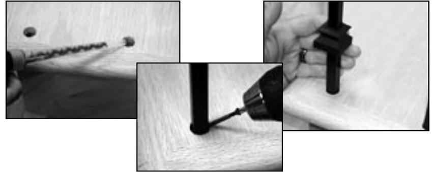
If top baluster collars are being used, place one on each baluster. Fill the holes in the handrail half full with construction adhesive. Position the handrail on top of the balusters and permanently secure the handrail to the newel posts. Secure every 6th baluster to the handrail with a flat head screw.
