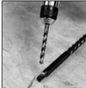
Fill tread holes half full with our two-part epoxy or construction adhesive. With a bottom collar on each baluster, place all balusters in position on the treads. Secure every 6th baluster with a flat head screw.
