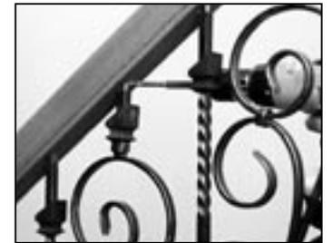
Any protruding epoxy or adhesive should be left to dry and can then be removed with a utility knife. Use an allen wrench to secure each top collar against the handrail and each bottom collar against the tread.
